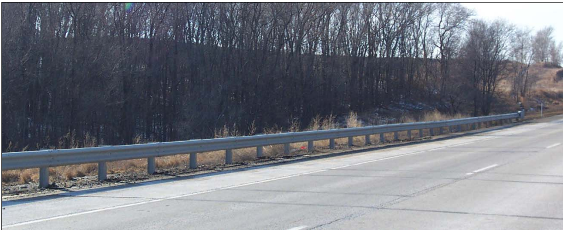
Figure 8. G4(1S) Strong Post Guardrail System.
