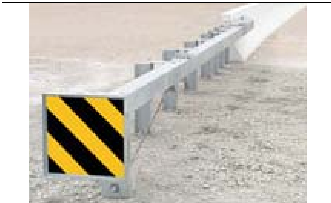
a) Installed BEAT-SSCC.
