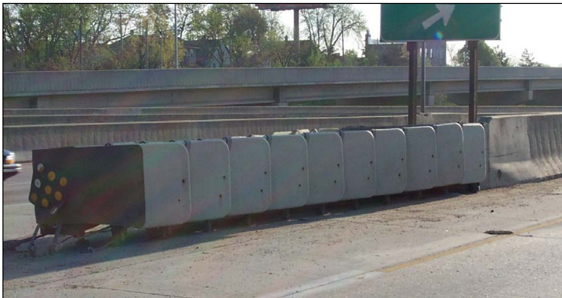
Figure 10. Hex-Foam Sandwich.
