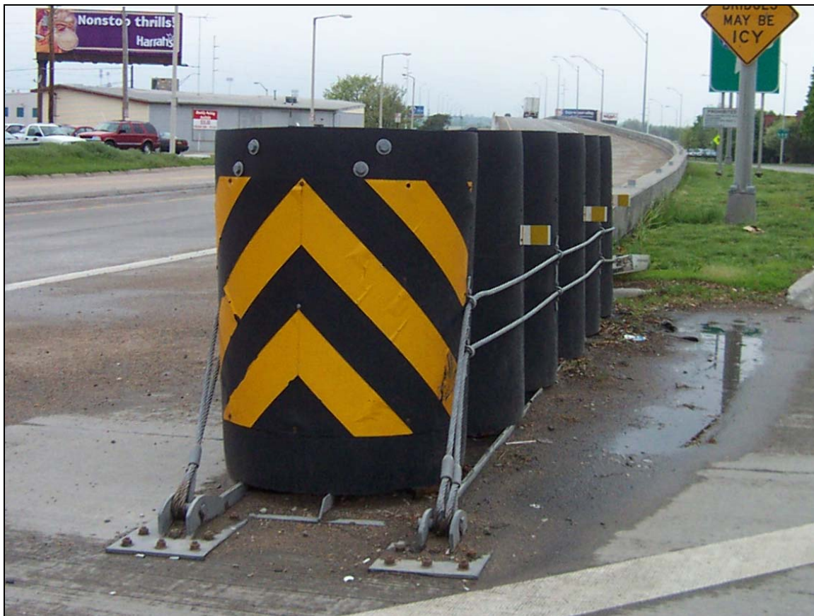
Figure 15. REACT 350.6, the Six-Bay REACT 350.
