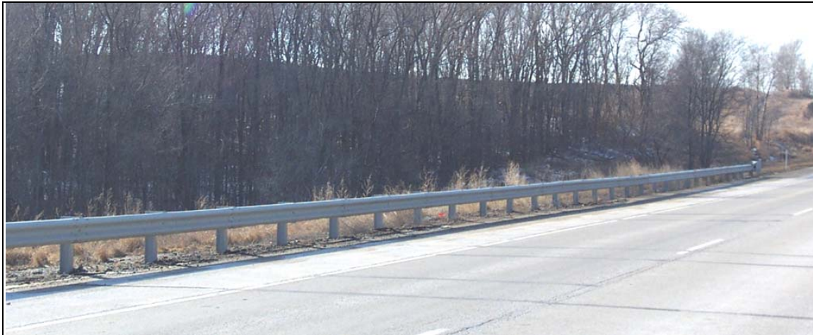
Figure 5. G4(1S) Strong Post Guardrail System.
